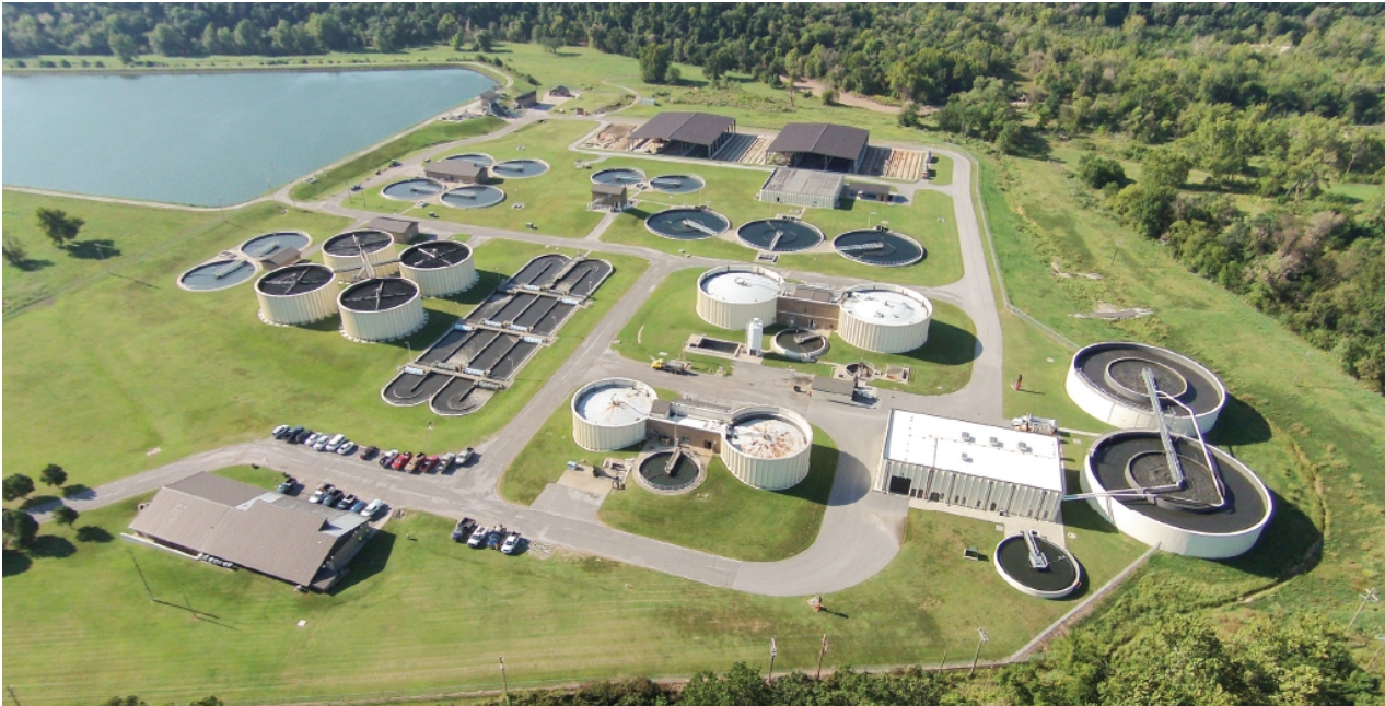
TURKEY CREEK WWTF
